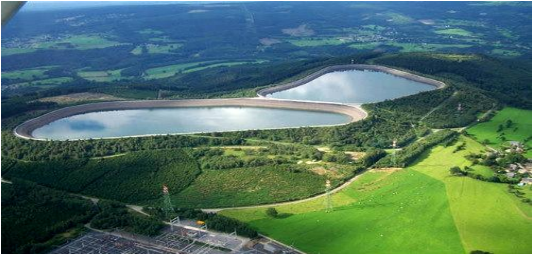
Coo-Trois-Ponts Pumped Storage Station, Belgium
