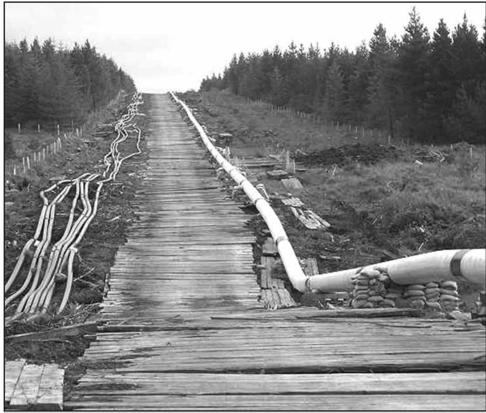
ROSSPORT FIVE: THE CORRIB OIL GAS PIPE LINE IN CO. MAYO
